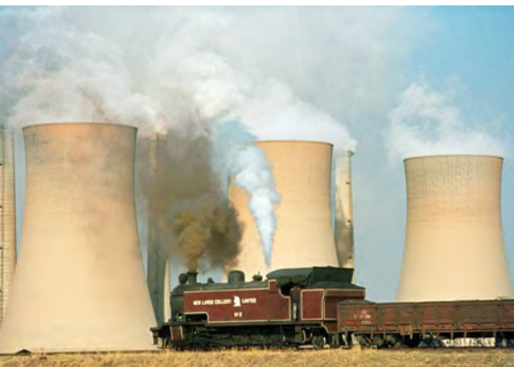
Figure 4.40 An example of a coal-fired power station
